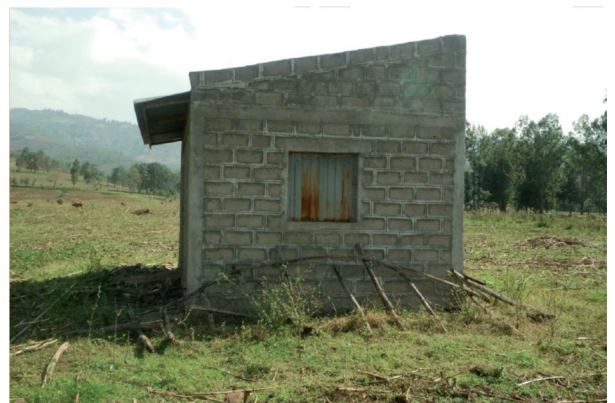
FIGURE 14 GENERATOR AND PUMP HOUSE
