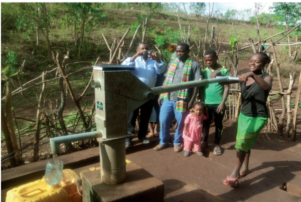
FIGURE 3 HANDPUMP (PROTECTED HAND-DUG WELL OR SHALLOW WELL)
