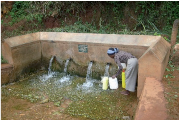
FIGURE 5 PROTECTED SPRING (NO LIFTING DEVICE)
