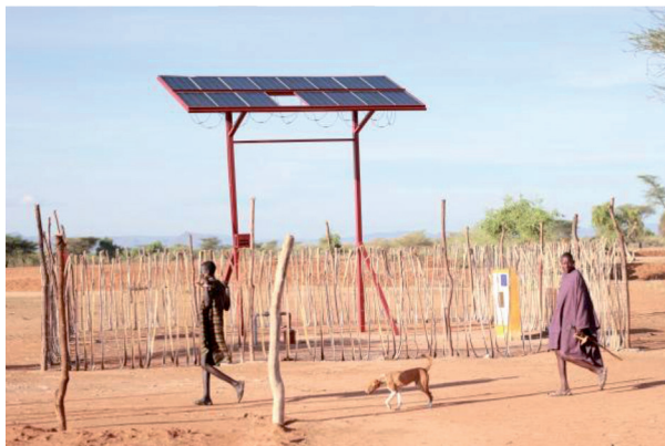
FIGURE 8 SOLAR WATER PUMP
