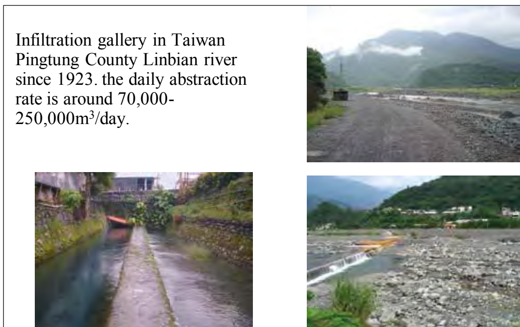
Figure 50: An infiltration gallery system in Pingtung, Taiwan.
