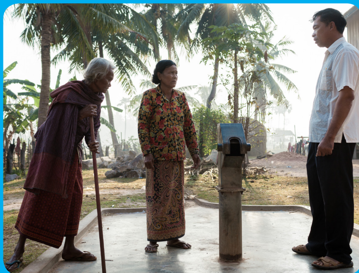
Ta Reach Village (Kampot). Mr. Oun (right), District Office of Rural Development, inspects a broken well. Photo: Thomas Cristofolletti / Ruom for SNV
