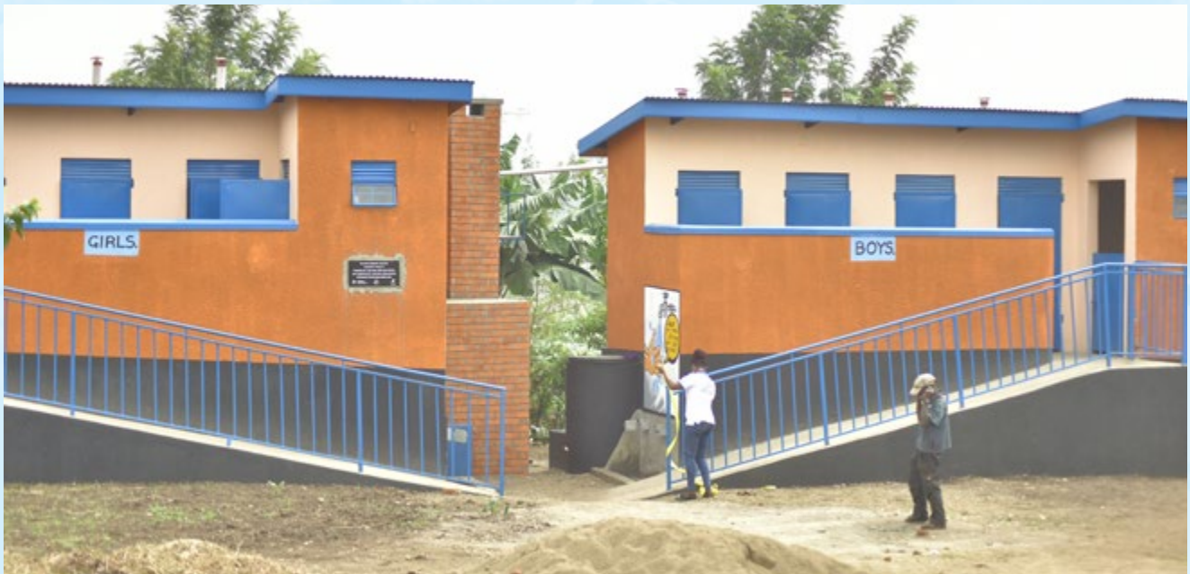
The new sanitation facility and rain water harvesting tank constructed by NRDl at Buhara Primary School, Kichwamba Sub-county.
