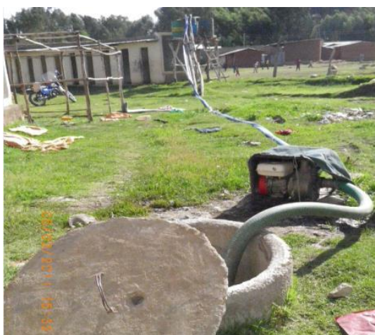
Figure 5. Hand dug well with plastic hose, diesel pump, 'barrel water tower' and shower rooms in Kombolcha district, Eastern Hararghe.
