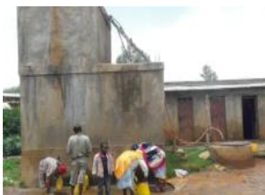
Figure 6. Hand dug well with engine pump, overhead masonry reservoir and shower rooms in Kombolcha district, Eastern Hararghe.
