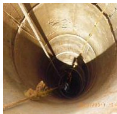
Figure 2. Well lined with concrete rings.
