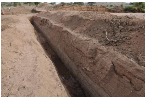
Figure 4. Excavated trench for sub-surface dam wall at Kenchera.
