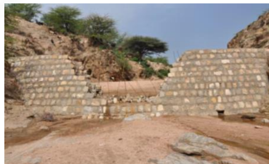
Figure 5. Partially completed sand dam at Gende Roba (August 2012).
