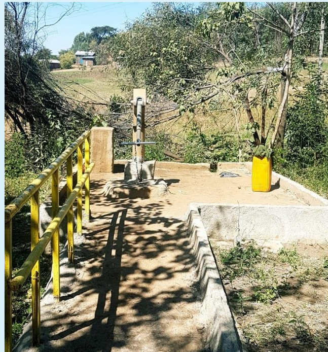
Rehabilitated and accessible hand dug well in Bahir Dar Zuria woreda, Amhara region.
