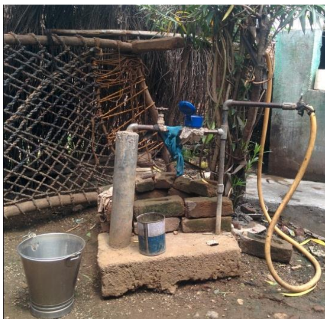
Photograph: a shared connection between two houses.
