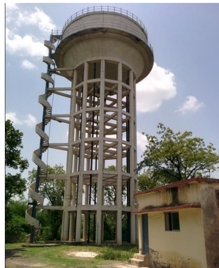
Photograph: Main Balancing Reservoirs and Elevated Service Reservoirs
