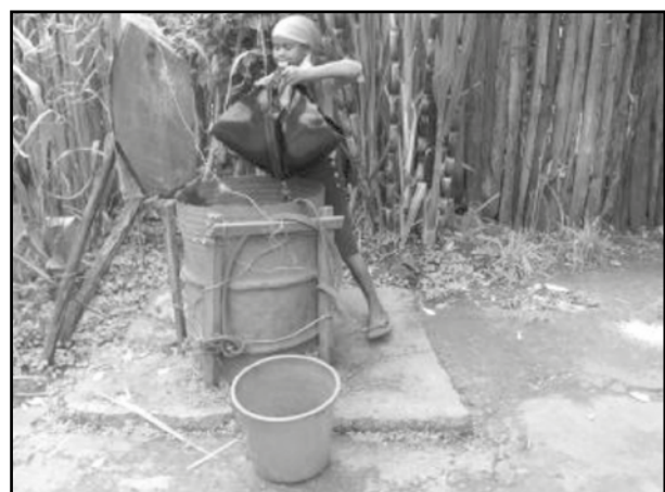
Figure 2.5 Semi protected well in Aleta Wendo (Photo: Sutton SWL Consultants)
