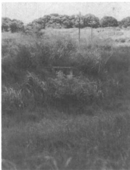
A partially overgrown malfunctioning waste stabilization pond.
