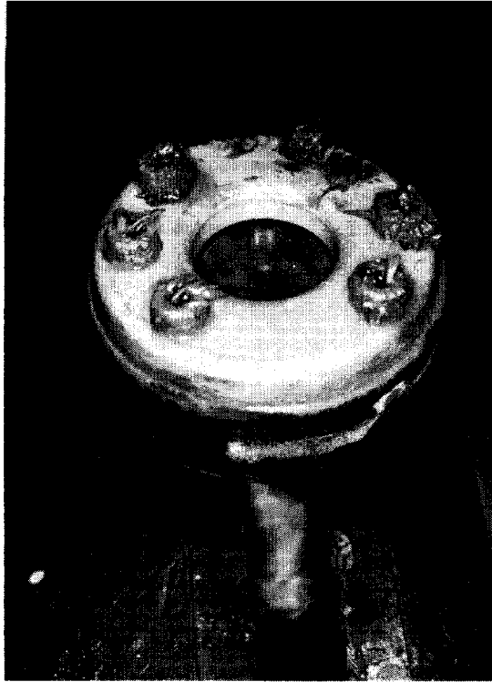
Original broken and corroded plunger fixing screws now replaced by stainless steel shouldered screws.
