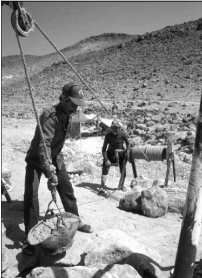
Clearing the qanat air shaft (Photo: Joshka Wessels)
