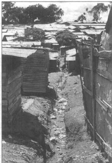
A Kibera latrine drains into the natural drainage channel.
