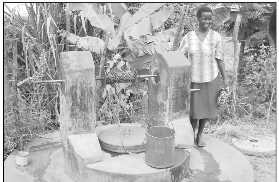
Mrs Toriwo of Makoni district in Zimbabwe funded construction of this upgraded family well herself
