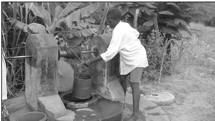
Upgraded wells such as this provide safe, sustainable drinking water close to the home
