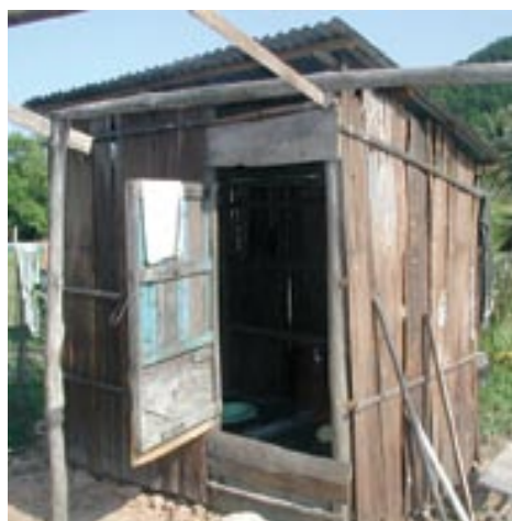
Using available wood, tin or plastic to make the toilet house
