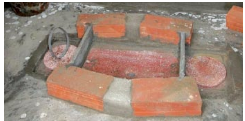
Installed Granito pan with two covered defecation holes
