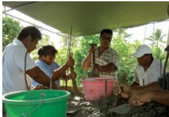
Trainees beginning to build the CT, Bonriki, Kiribati
