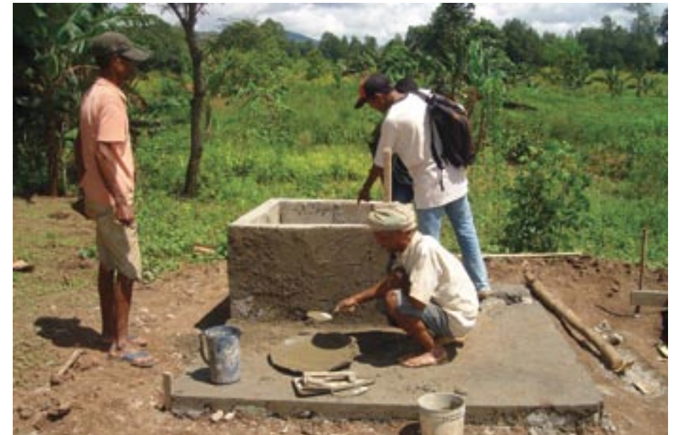
Local masons constructing a latrine
