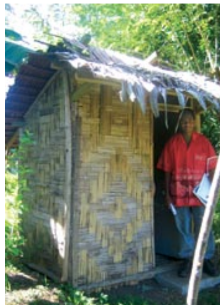
A functioning VIP latrine
