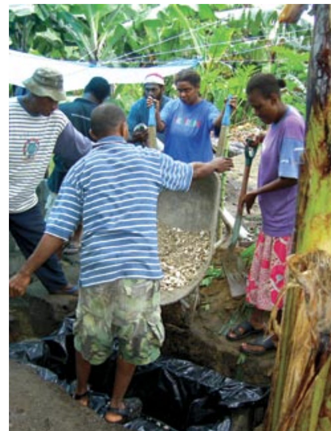
Trainees pouring aggregate into evapotranspiration trench, Vanuatu
