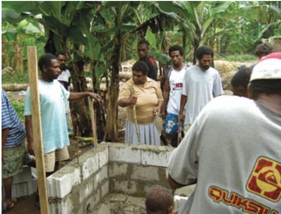
Trainees building composting chamber, Vanuatu
