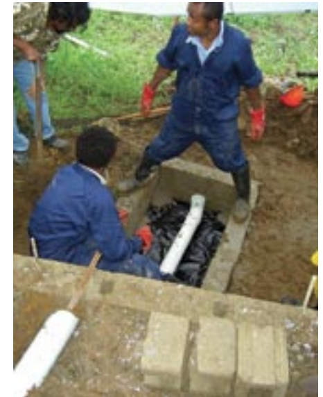
Hands-on community training to build drainage trench for composting toilet
