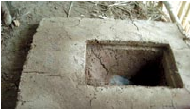
A squatting pan made from local materials
