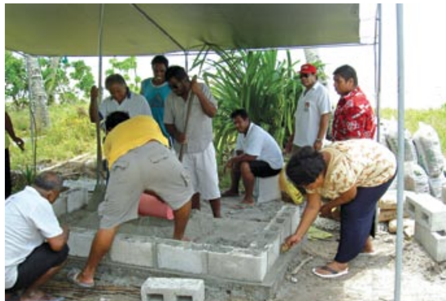
Trainees pouring slab for toilet room floor in Bonriki, Kiribati
