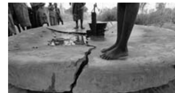
In many developing countries broken water supplies are common. Without the management infrastructure in place to maintain them it is common for water facilities to break down. The water collected from this pump in Malawi will now be polluted as the top is no longer sealed.
