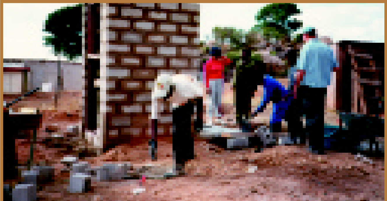
Constructing VIP latrine superstructures.
