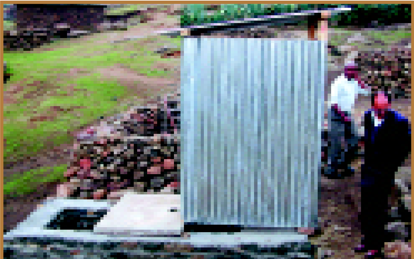
VIP latrine under construction in Lesotho.
