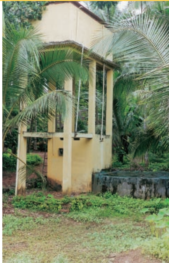
A water tank constructed under a private drinking water scheme
