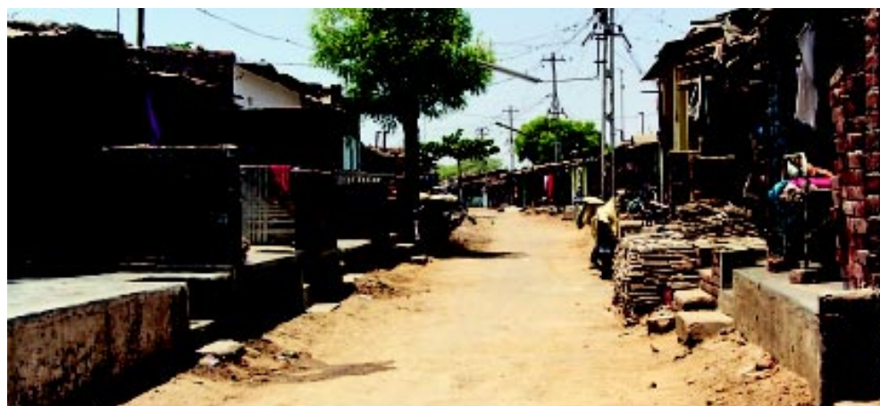
Wide Inter-connecting roads of Ramdevnagar following the upgradation
