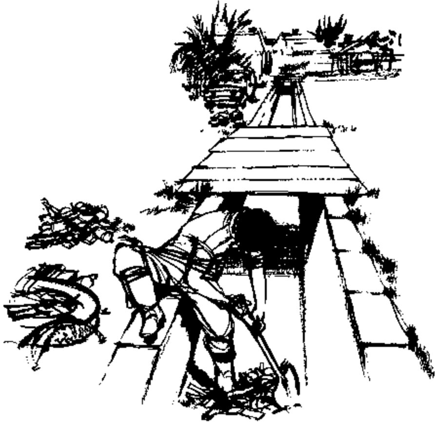
Fig. 6.10. Regular cleaning of drains is needed to avoid fly breeding in accumulations of garbage.
