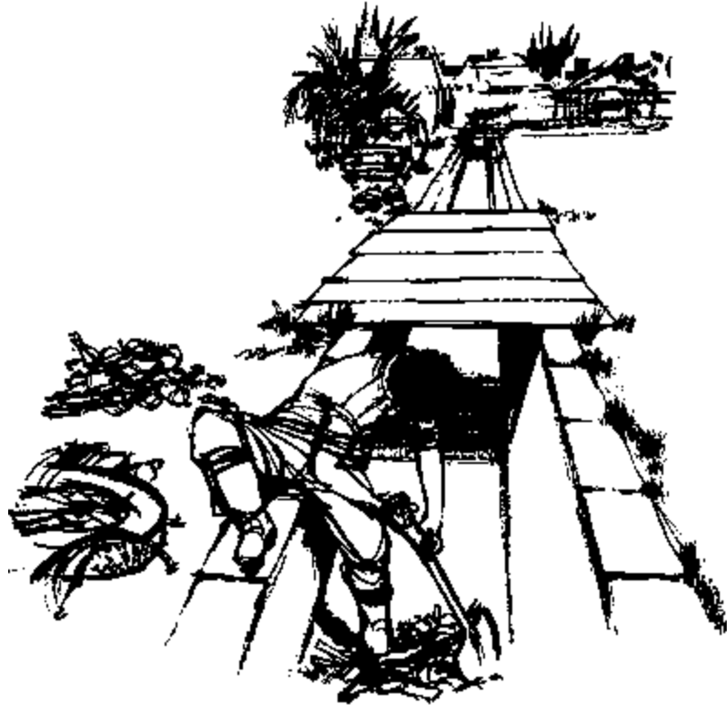
Fig. 1.128. Dirt, debris and other obstacles in drainage systems should be removed to allow the water to flow freely.
