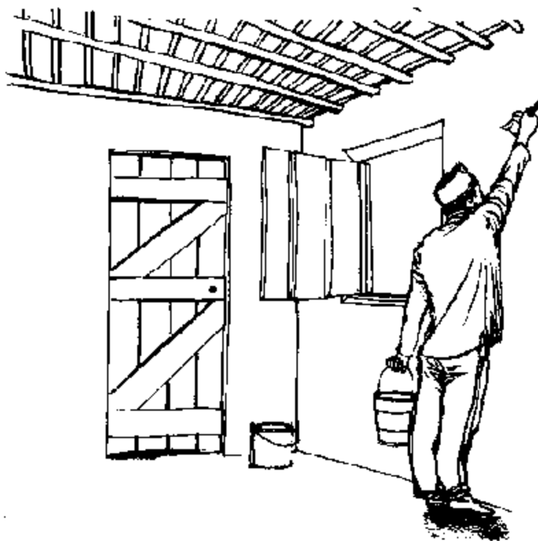
Fig. 3.11. Slow-release insecticidal paints are suitable for brush-on application.
