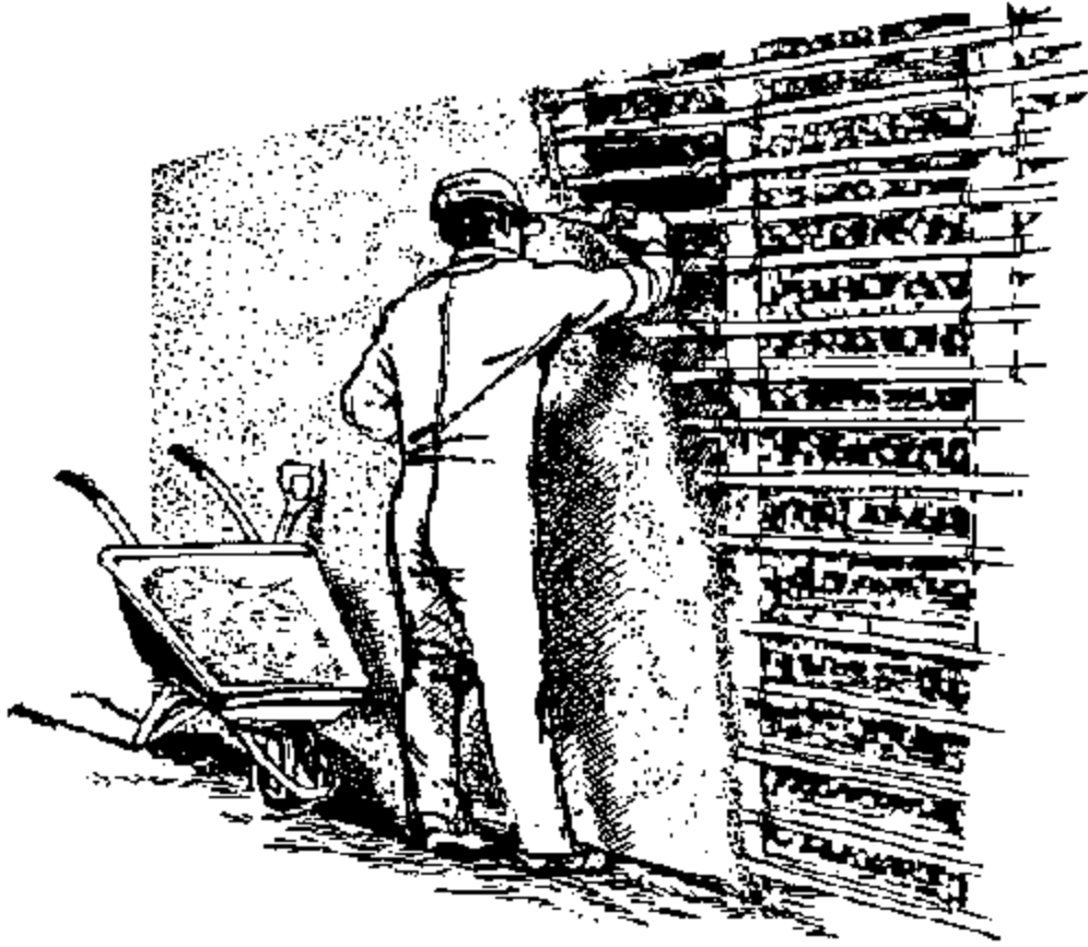
Fig. 3.16. Resting places in walls can be filled with plaster, which can be applied by hand and smoothed by hand or with a trowel.
