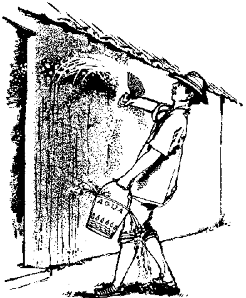
Fig. 3.17. The surface has to be wetted before the next layer of plaster is applied, in order to improve adherence and prevent cracking caused by excessively rapid drying.
