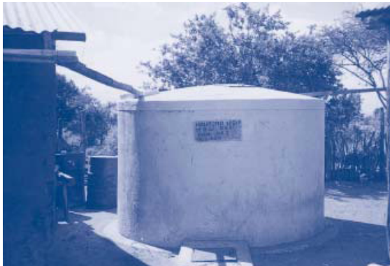
Figure 1.19 Simple roof catchment and storage. Source: IRC.
