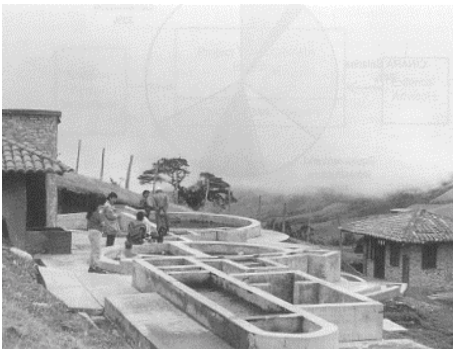
Figure 5: The MSF plant in Paispamba, Cauca, Colombia, one of the demonstration systems
