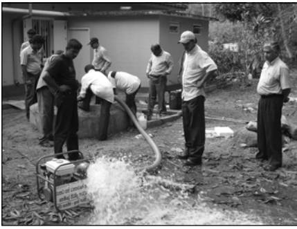
Well cleaning after the tsunami , demonstrating what not to do, i.e. discharge saline well water next to the well
