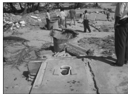
Devastation of wells and pit latrines as a consequence of the tsunami . Note that wells and pit latrines were often sited quite close to each other.
