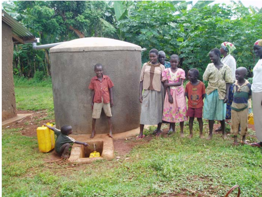
Domestic Roofwater harvesting in Kaproron Sub-county, Kapchorwa District
