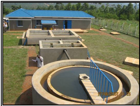
Sembabule water treatment works
