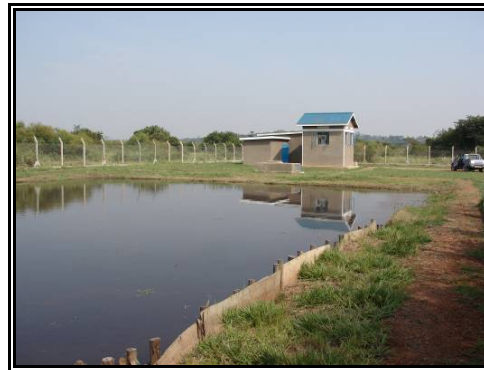
Sembabule water intake works
