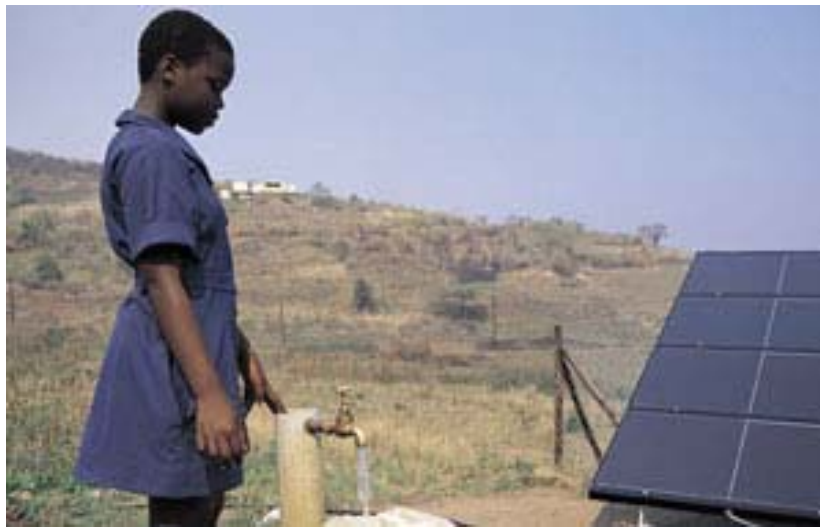
A school girl fetching water from a Solar Powered Piped Water System in Nebbi District
