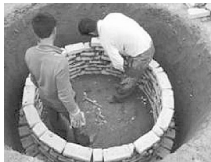
UNICEF is training local masons in the construction of sanitary toilets
