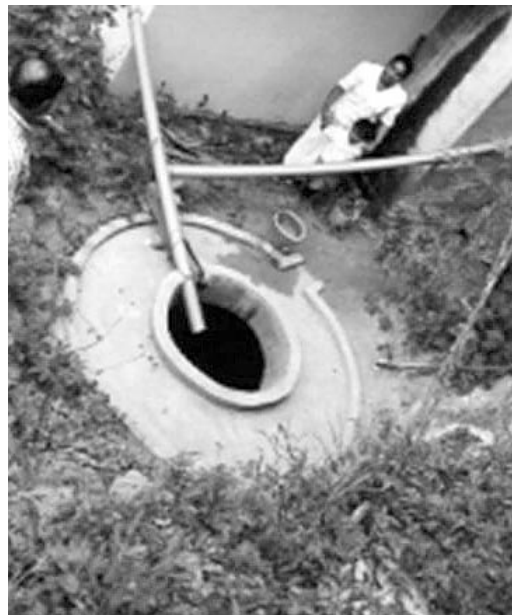
Underground domed brick tank storing roofwater for household use: capacity 5,000 litres
