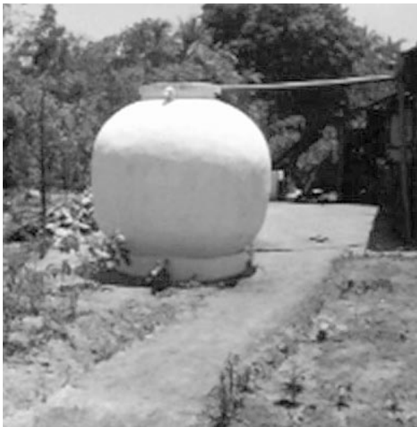
Surface ferrocement tank storing roofwater for household use and home gardening: capacity 5,000 litres
