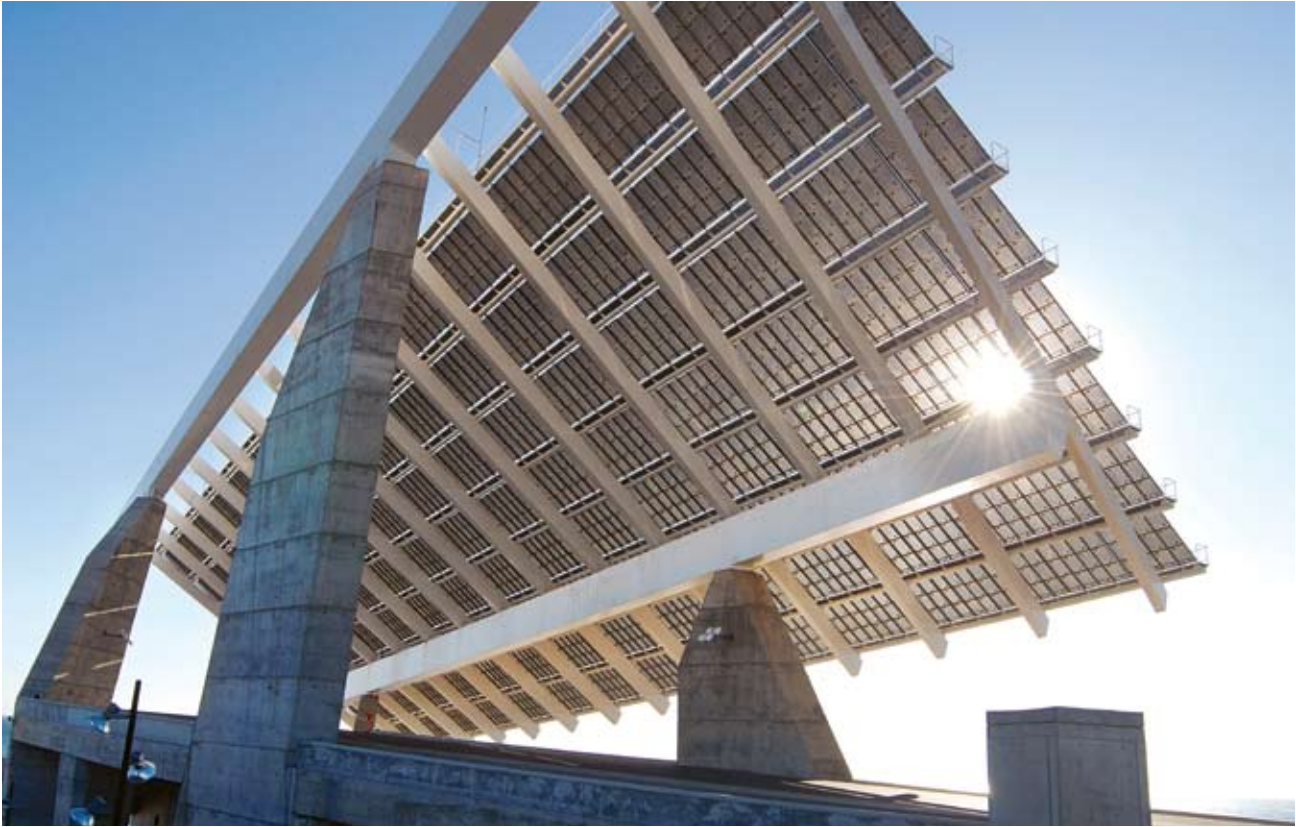
▲ Solar panel installation in Barcelona, Spain ©Snezana Negovanovic/iStockphoto
