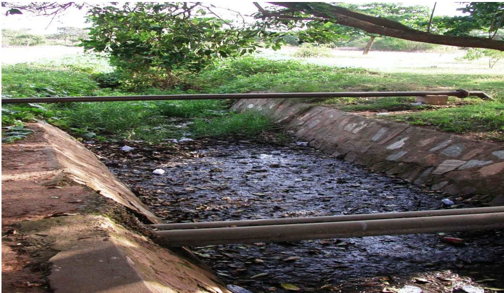
Figure 4-6 Typical storm water drain in the city
