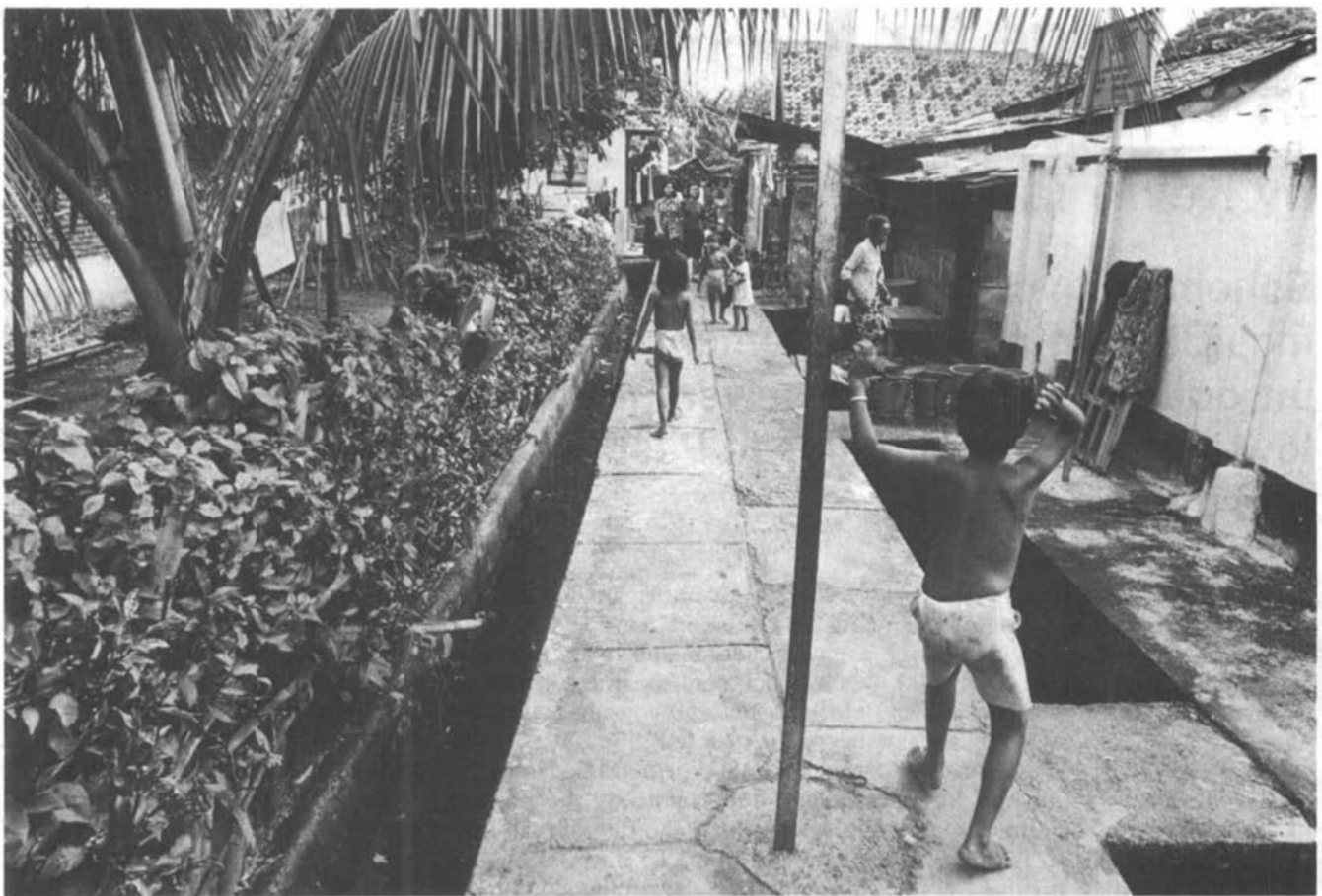
A concrete path improves this housing area but the open drain remains.
