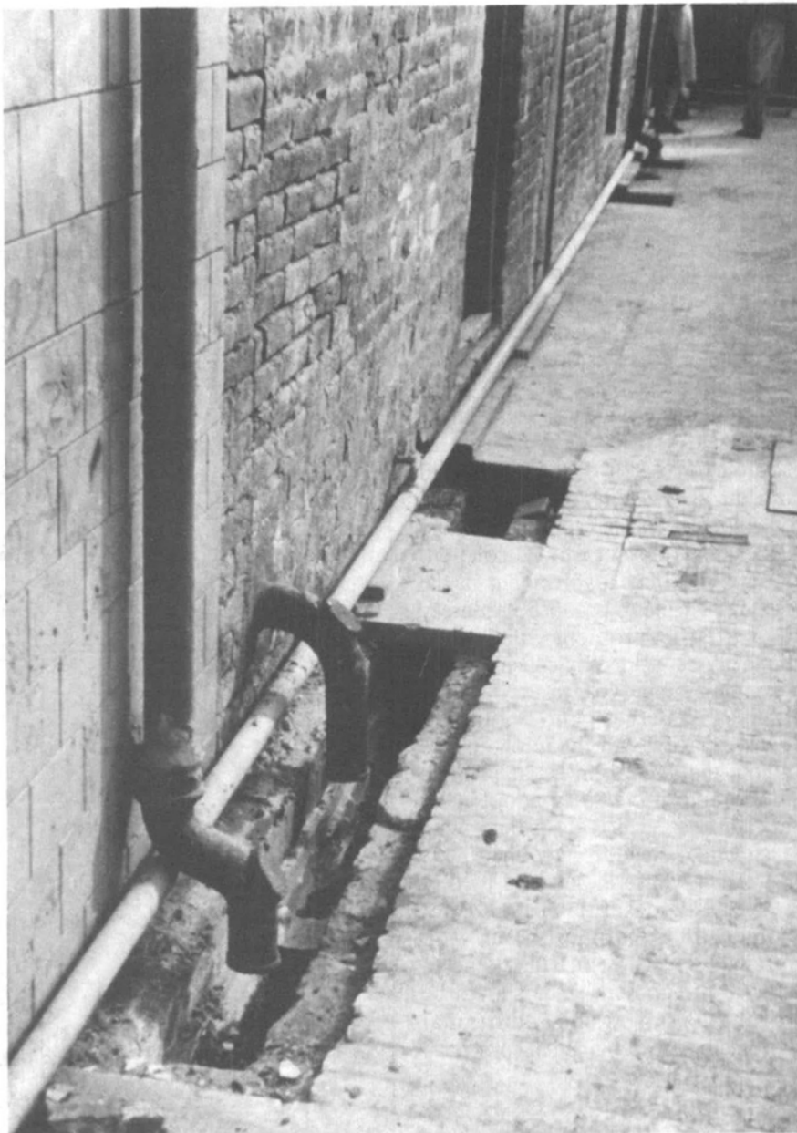
This side drain in North-east Lahore has its connecting pipes in place, but is still waiting for cover slabs.
