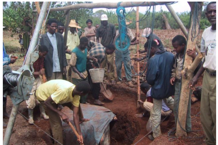
Figure 5 Self help well construction in Ethiopia
