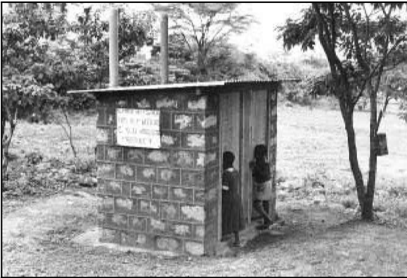
New school latrines in Kenya
