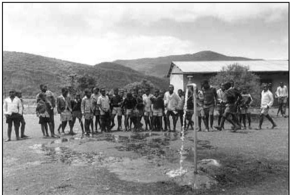
Rural schoolchildren witness the first flow of water from piping laid by the Rural Advice Centre, a development NGO – the area has a high incidence of bilharzia (Mafefe, Northern Transvaal, South Africa).
