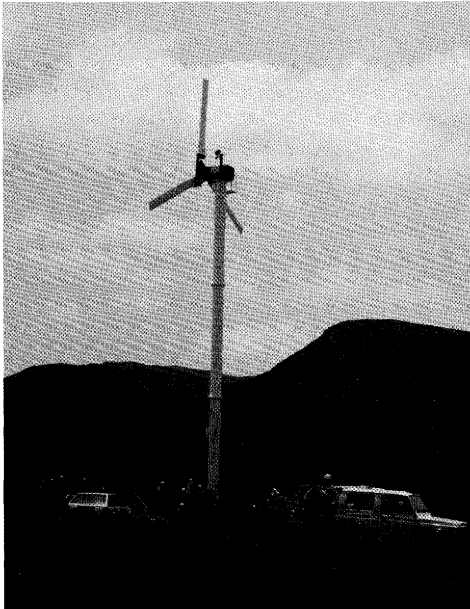
Wind electric pumping system (WEPS) on Cape Verde. A Lagerwey wind turbine of 10.6 m rotor diameter is installed on an 'achada', well exposed to the wind, and drives an electric deep-well pump in the valley. Note the hydraulic jack at the tower base for erection without the need for a crane.
