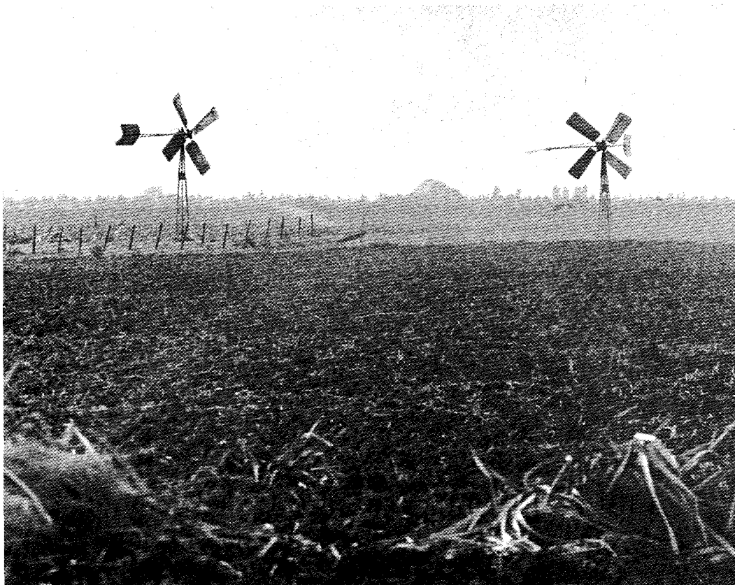
Bosman wind pump driving a centrifugal pump. Thousands are in use in the Netherlands to pump water from the drainage canals of the polder over heights of 1 m or less.
