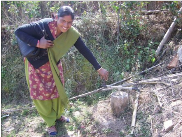
Offtake taps for irrigation purpose
