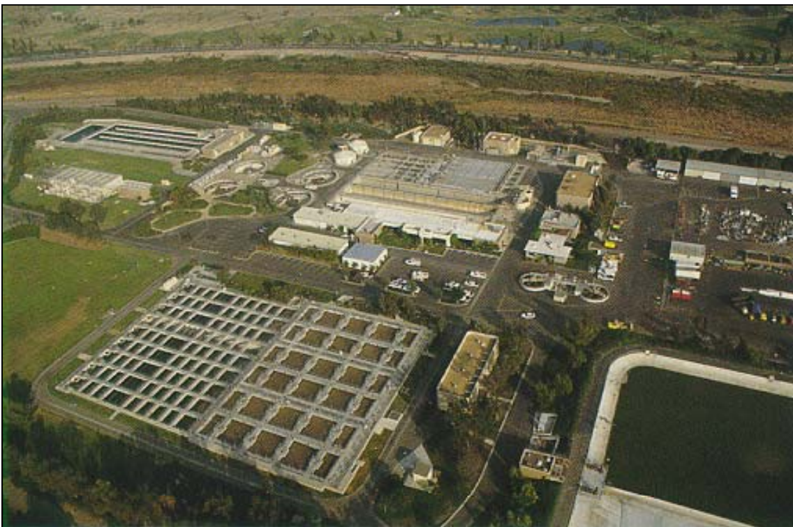
Figure 11: Michelson Water Reclamation Plant (Irvine Ranch Water District, 2001)
