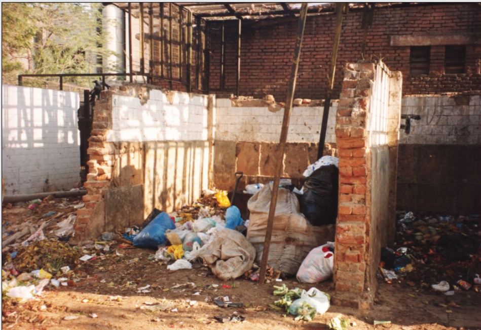
Poorly maintained transfer point in Delhi suburb
