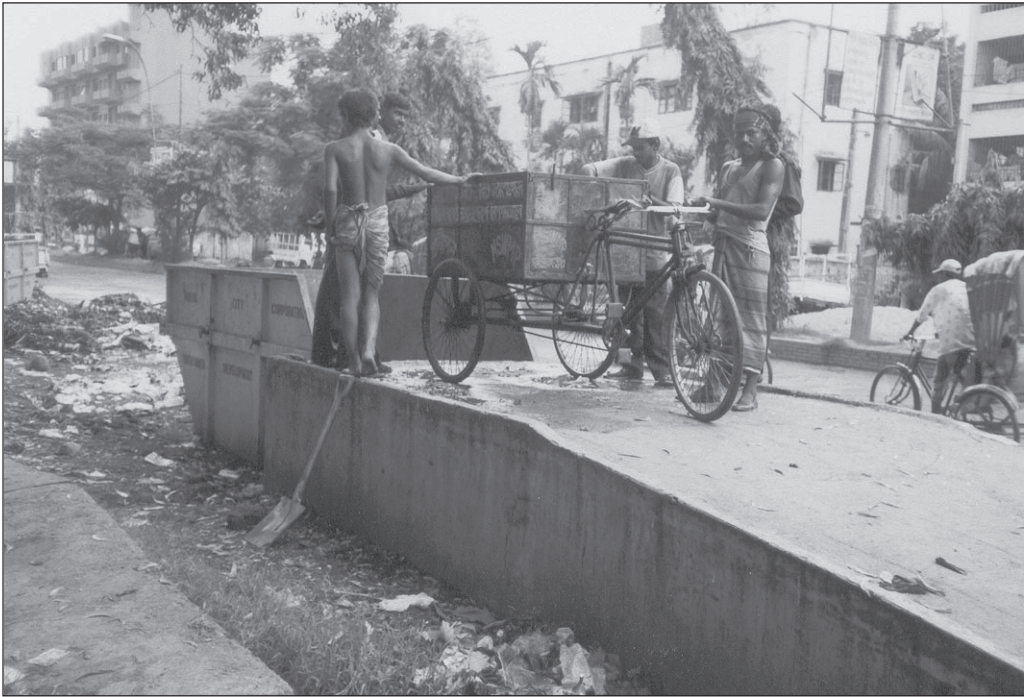
Ramp transfer system in Khulna, Bangladesh
