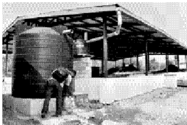
Photograph 6.1: Rainwater harvesting system at the co-composting pilot plant in Kumasi, Ghana. The small "first flush tank", behind the main tank, collects the first incoming rainwater, diverting dust and dirt from the roof. (Sandec)
