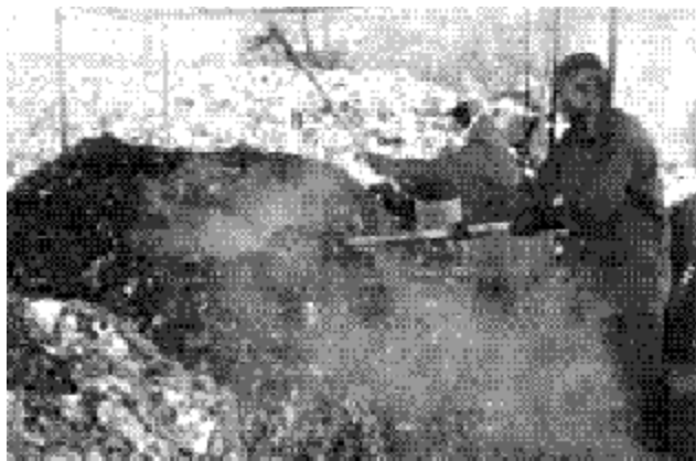
Photograph 7.7: The windrow is turned weekly to improve the aeration of the pile. The steam indicates the high temperature and water loss during the composting process (Waste Concern, Bangladesh)
