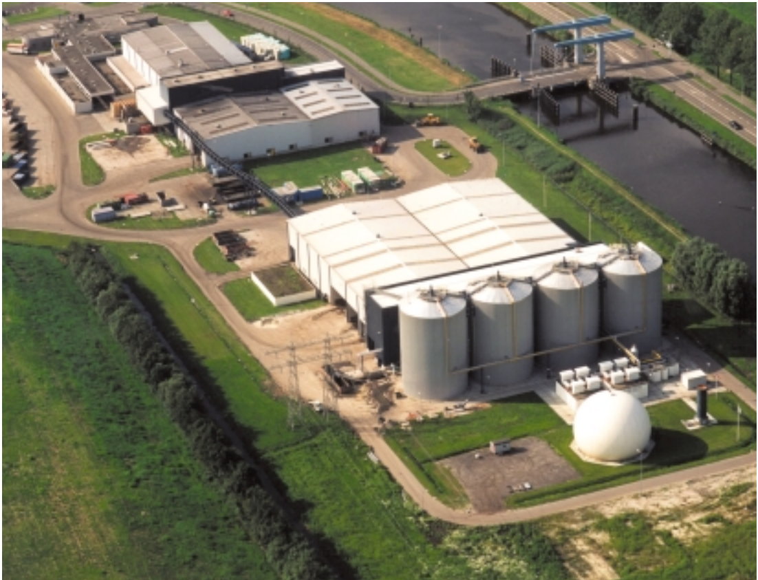
Figure 11. Vagron plant (Groningen) for separation and digestion of the organic fraction of MSW. Photo by courtesy of Vagron BV.
