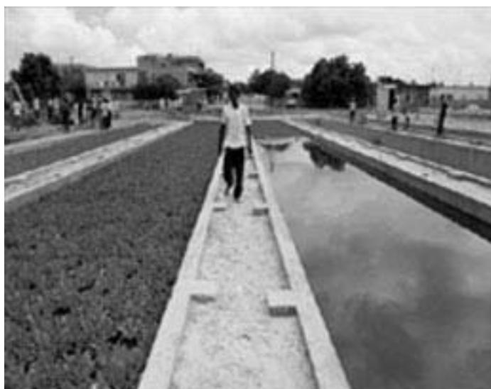
Community wastewater treatment plant using aquatic plants (Dakar, Senegal)
