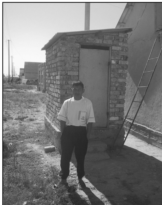
This Ventilated Improved Pit Latrine (VIP) in Kyrgyzstan was constructed by the house owner, based on his observations of latrines seen in rural areas.
