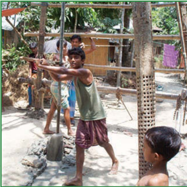
Drilling to depths of over 300 meters can be done using manual methods
