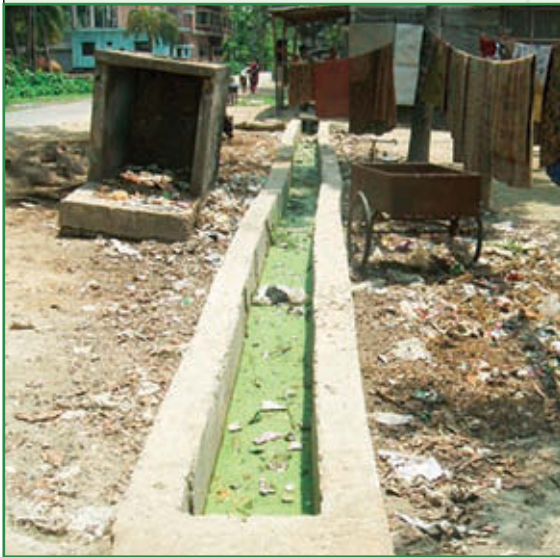
Dustbins and drains are often poorly maintained
