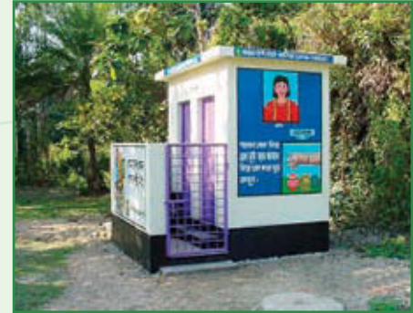
Separate toilets are constructed for girl students with colorful health messages
