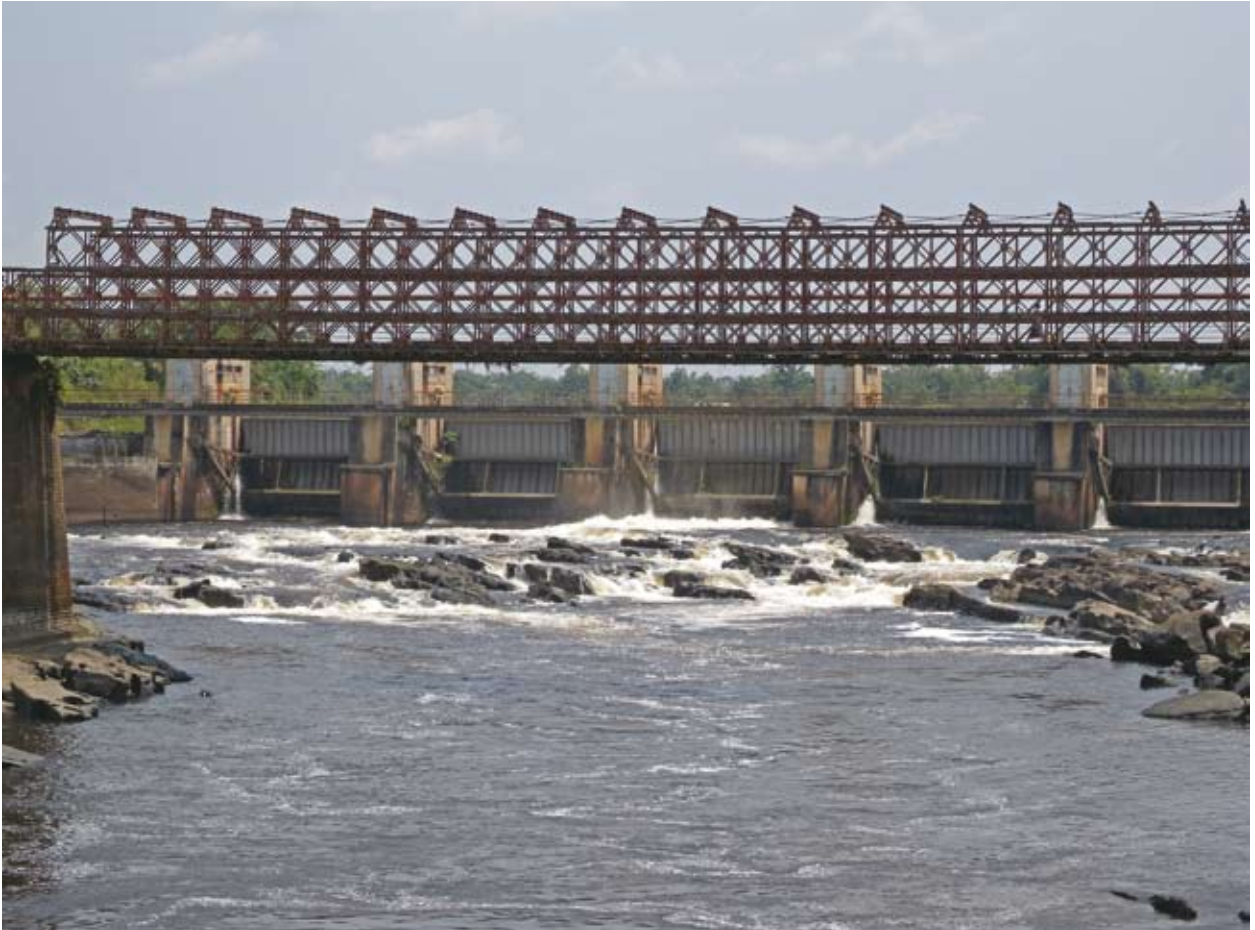
Tshopo hydroelectric plant in Kisangani, Orientale Province, is one of the DRC's many run-of-the river schemes having a limited environmental footprint
