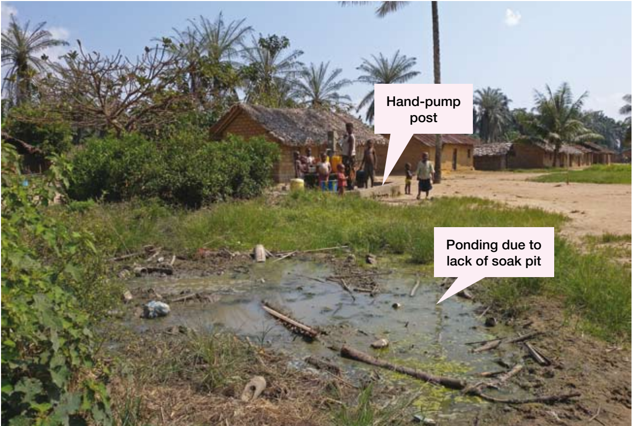
Without a drainage canal to remove excess water produced from hand-pumps, resulting stagnant pools may become breeding grounds for infectious diseases. (Bilundu Village, Maniema Province)
