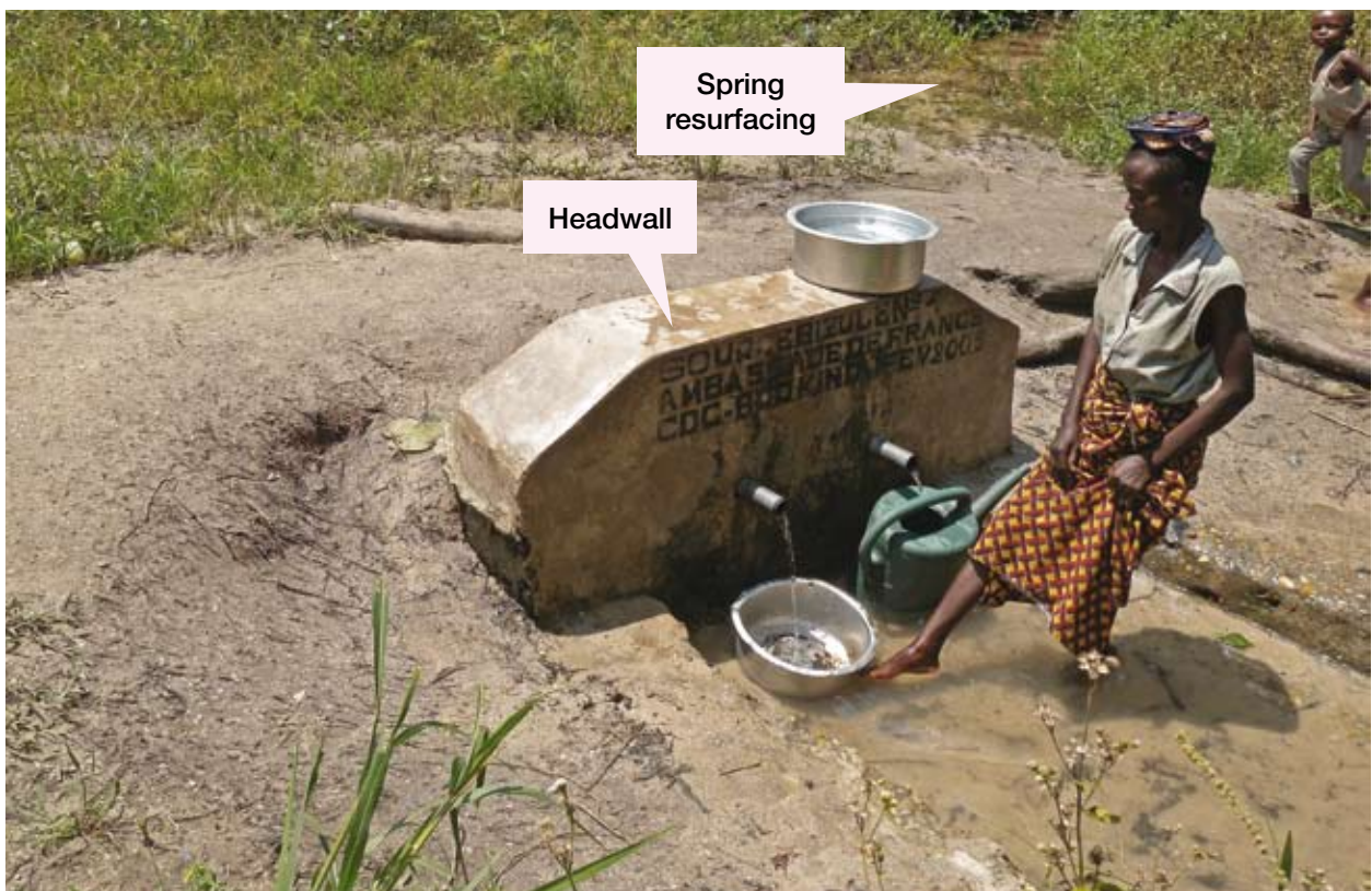
Retaining walls are simple alternatives to spring boxes, but even such basic structures require a minimum level of maintenance and site protection. As the headwall is not properly positioned, back-pressure has caused the spring eye to move and re-emerge to the right
