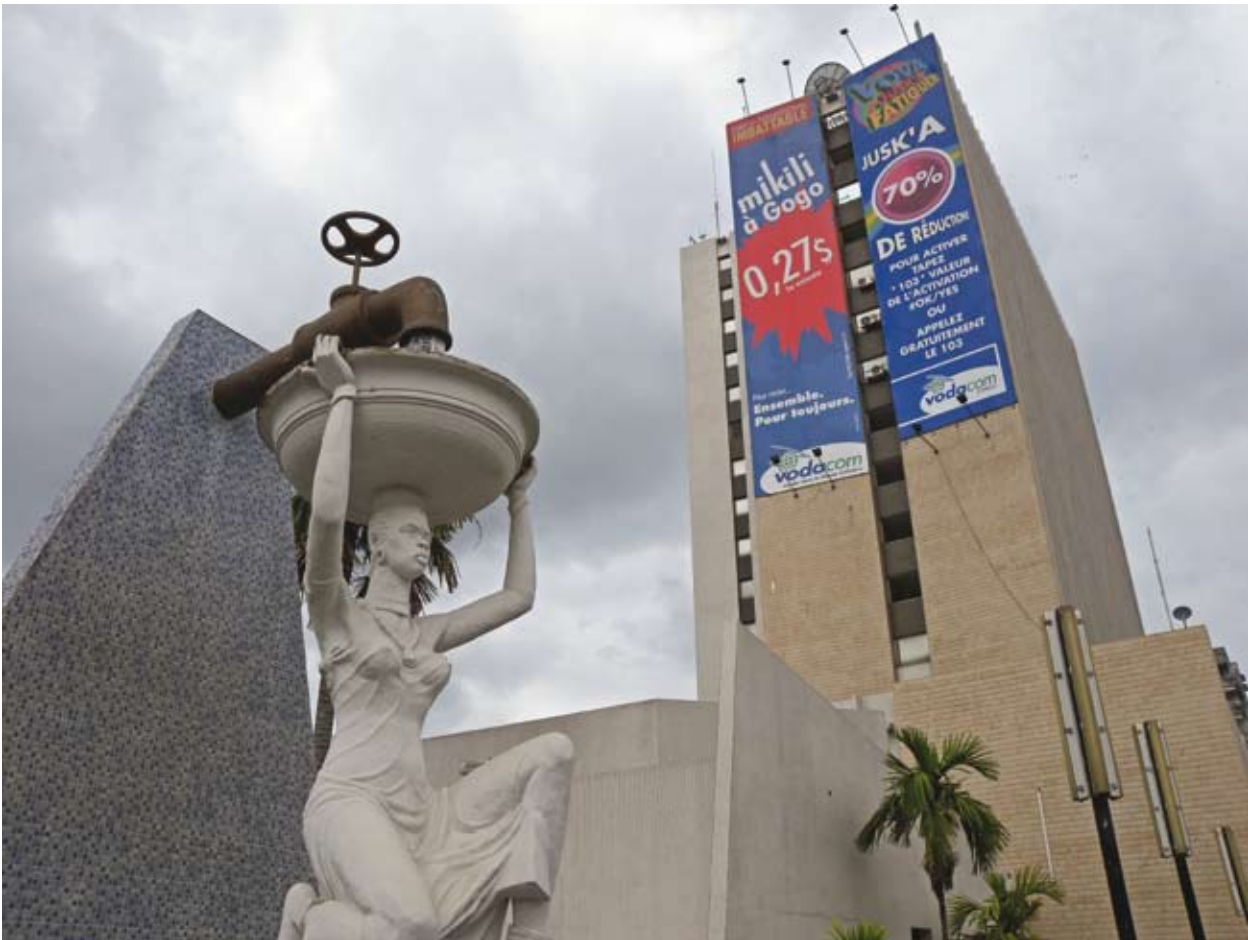
Up until the early 1990s, the REGIDESO was reputed to be one of the most successful public water utilities in Africa. REGIDESO headquarters on the Boulevard du 30 Juin in Kinshasa
