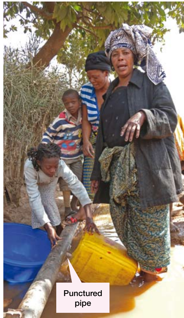
Local residents queuing in the Cité Musonoie in Kolwezi to draw water from breaches in the water pipeline (Katanga Province)
