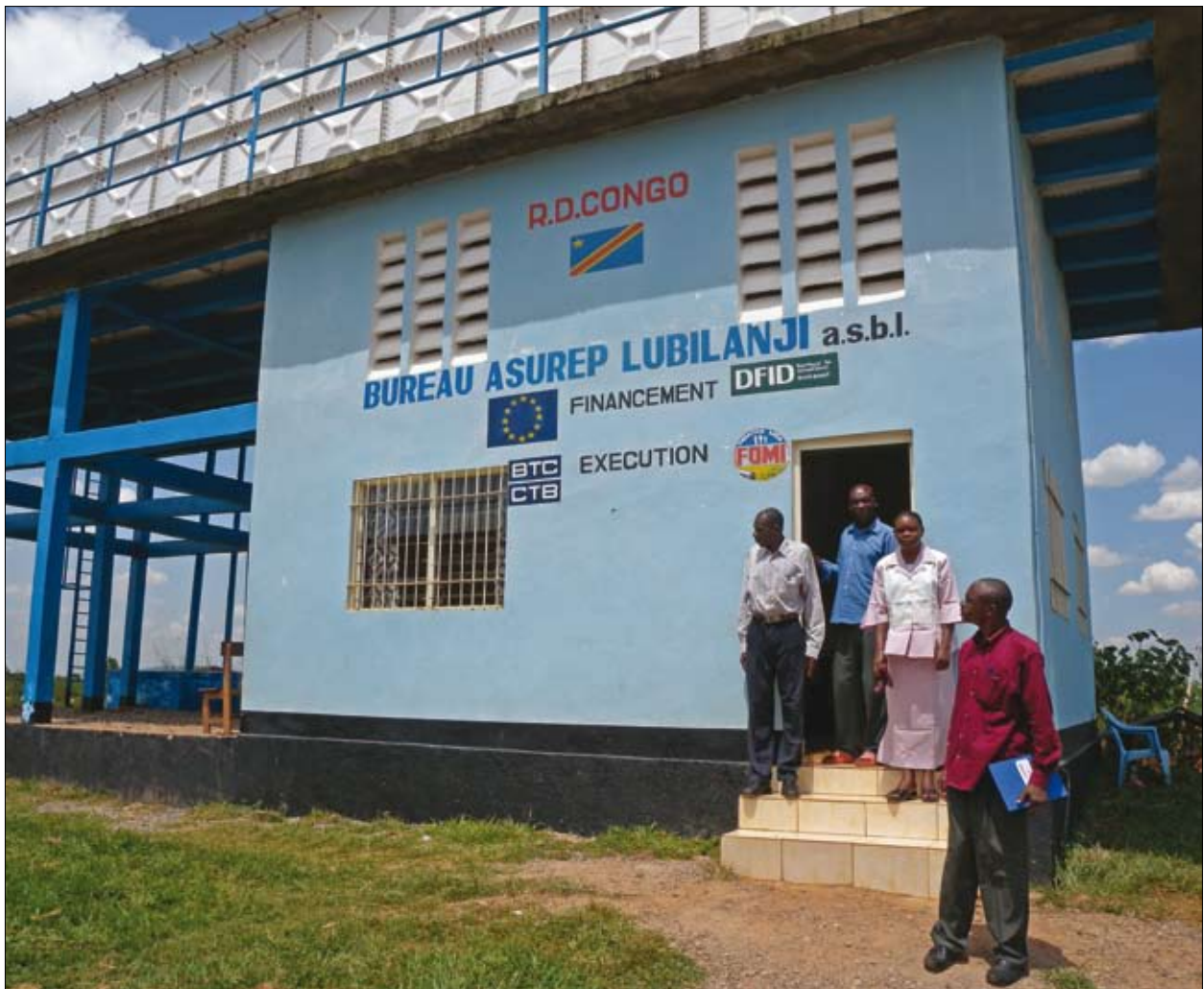
Newly constructed office of the Lubilanji Water User Association in Mbuji-Mayi, Kasai Orientale. Following a breakage in REGIDESO's pipeline in February 2010, this was one of the few sources of potable water in the DRC's third largest city
