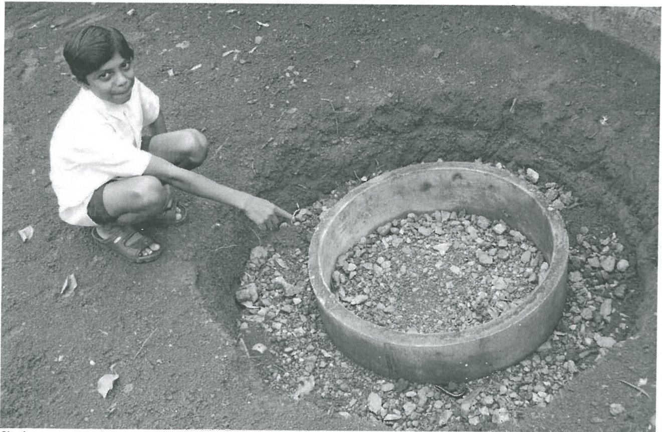
Simple groundwater recharge to augment open wells.
