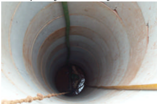
Community working inside a hand-dug well
