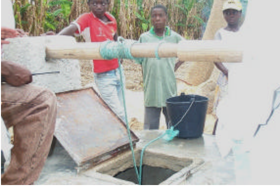
Construction of a spring protection
