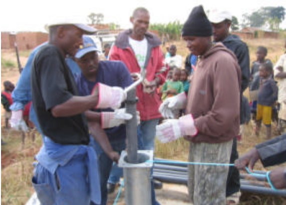
Installation of a borehole's hand pump
