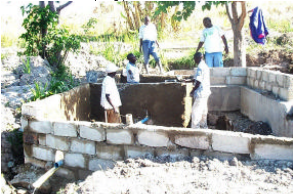
Community collecting water from a hand-dug well
