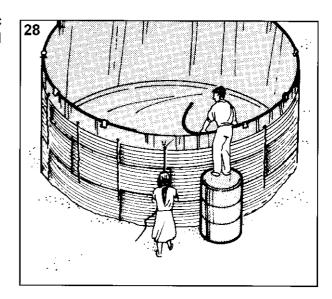
**29.** When the tank is complete, the liner seams should hang vertically and not stretch when the floor/wall seam is pushed into the corner.
