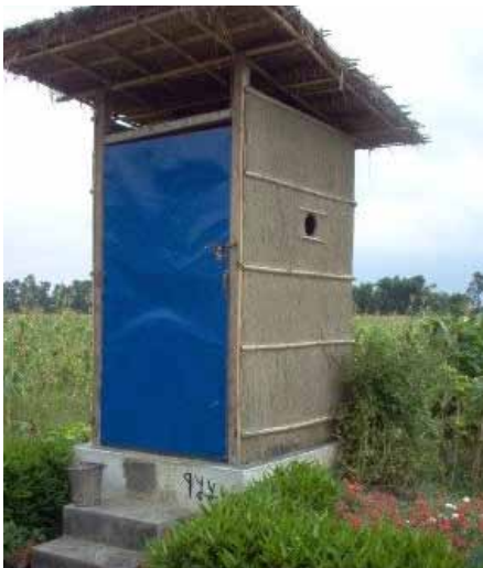
FIGURE 3.6 New Toilets from UN-HABITAT Project and New Tap Connection
