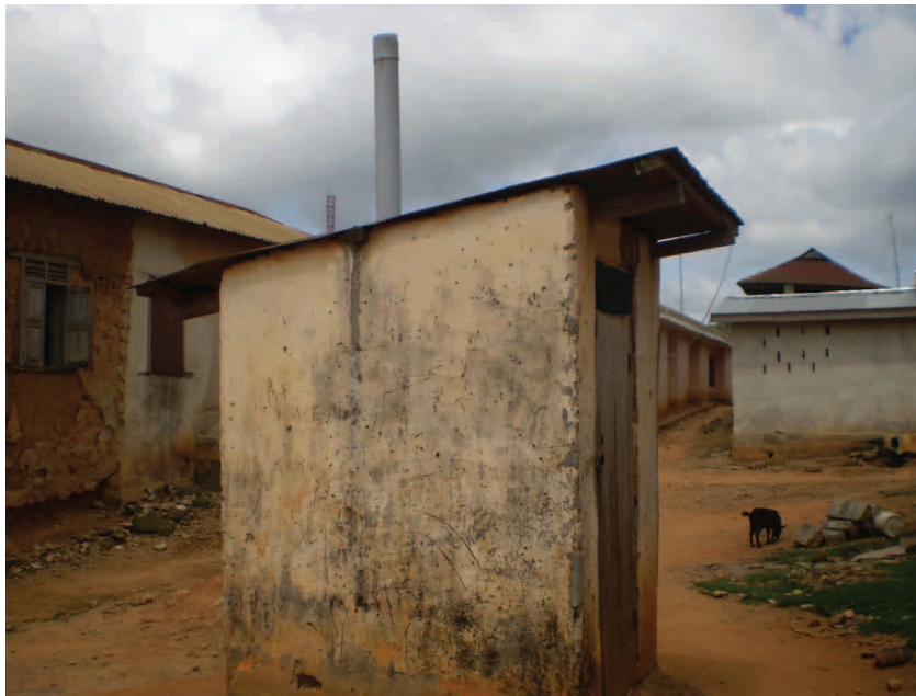
Plate 1: A typical VIP latrine in a small town
