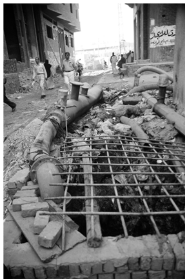
Inlet structure for temporary pump station in Ezbet el Nawar
