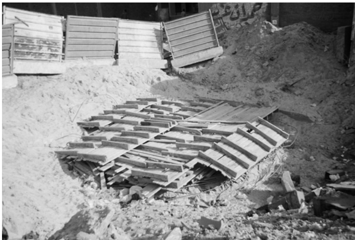
Incomplete CWO pump station and force-main system
