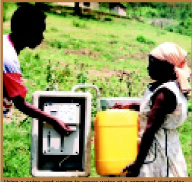
Using a swipe-card system to access water at a communal stand-pipe.
