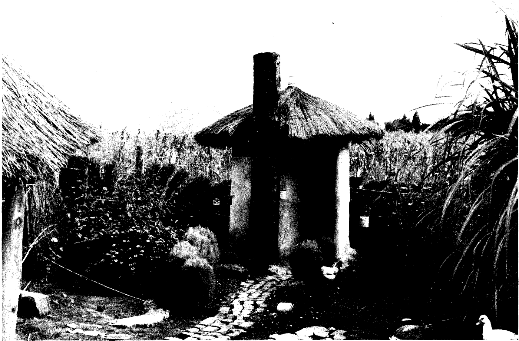
Figure 10: Mud and wattle spiral VIP latrine.
