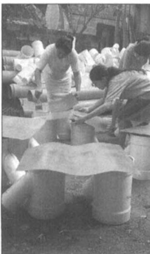
Community water-pipe construction.
