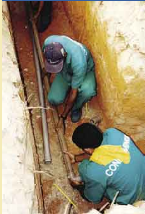
Installation of the Public Water Network, Parauapebas
