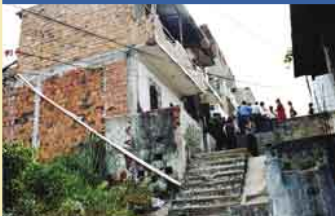
Steep Change of Condominial Branch Level (pipe attached to wall), Sao Caetano, Salvador de Bahia
