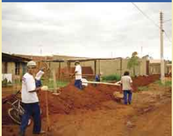
Excavation works, Brasilia
