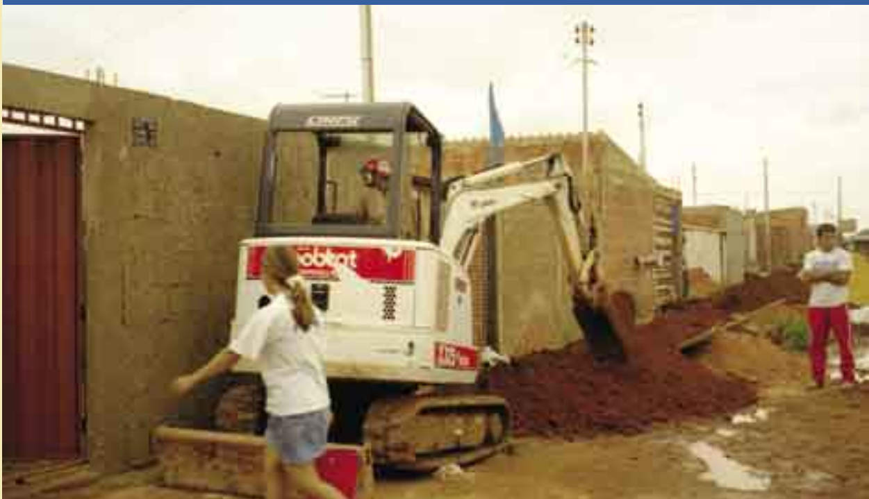
Excavation for the Public Network, Brasilia
