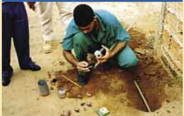
Installation of micro-meter in household connection, Parauapebas
